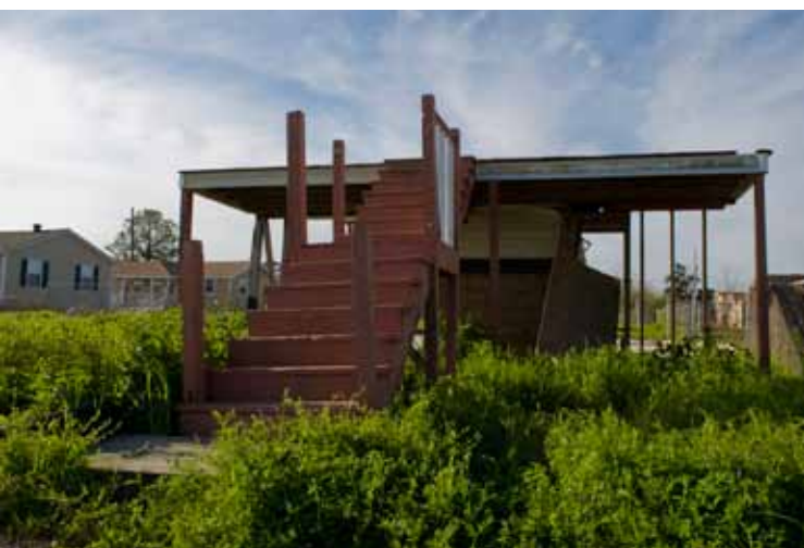
Nearly five years after Hurricane Katrina struck the Gulf Coast, crumbling buildings and empty foundations can still be found throughout the 9th Ward in New Orleans in 2010.
