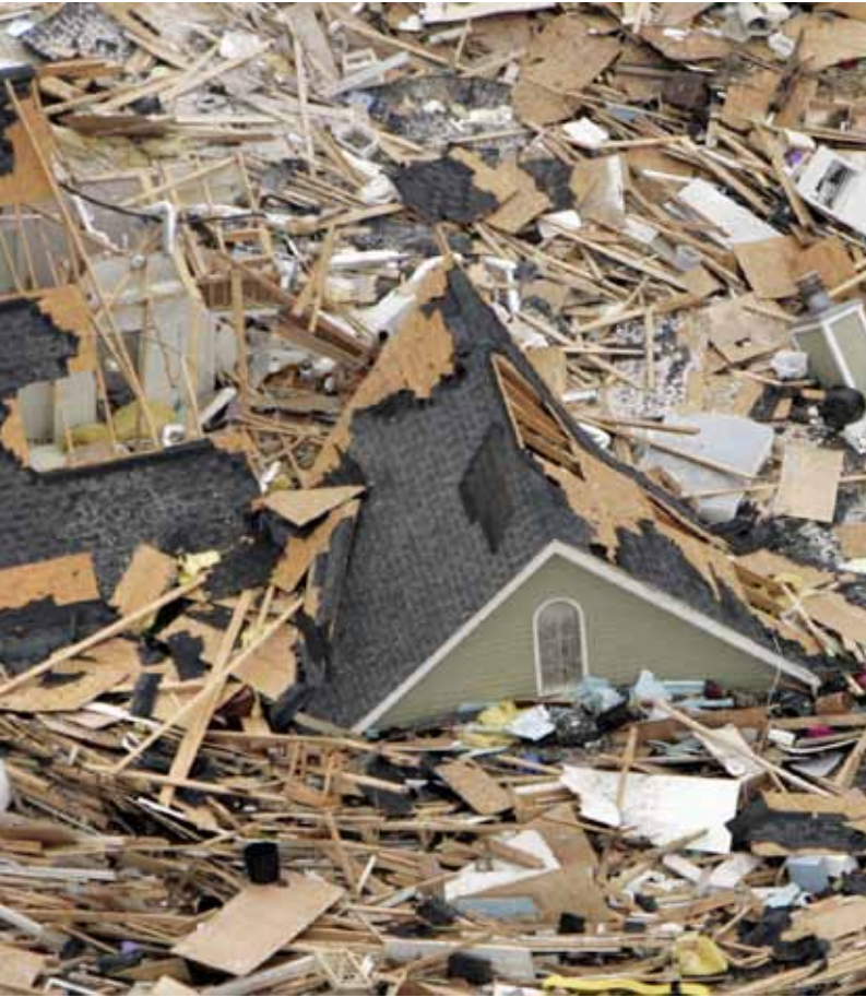
Rubble surrounds a house in an aerial view of damage from Hurricane Katrina in Long Beach, Mississippi.
